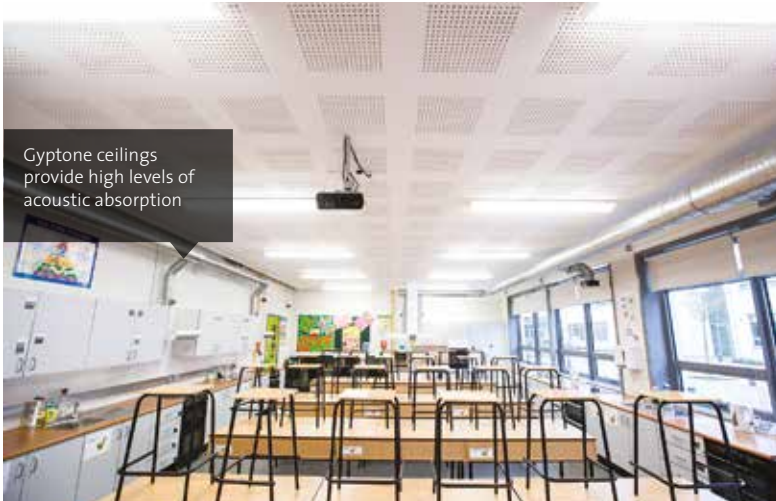
Gyproc CasoLine MF framing facilitates change of level details to enhance the lighting strategy
